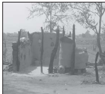
Photo 3. After fire in a thatched roofed building in Kapilbastu
