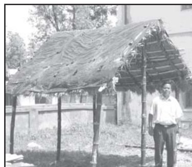
Photo 4: Showing the fire resistant technology
