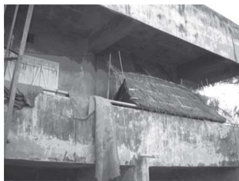
Cyclone Shelter occupied by local people at Moheshkhali; Picture 11 th November 2005.
